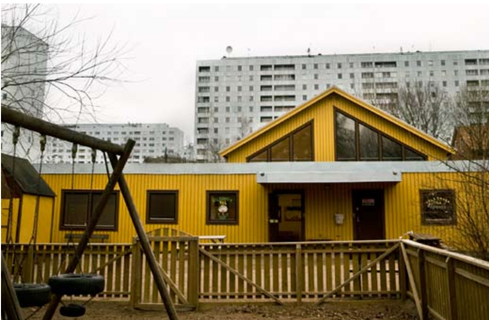
Late afternoon and everybody has left. The exterior of a quite typical Swedish daycare centre – a one-storeyed wooden building,, surrounded by a low fence.
